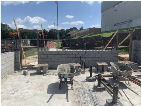
FD- Door frames set in preparation to close in and grout pour
